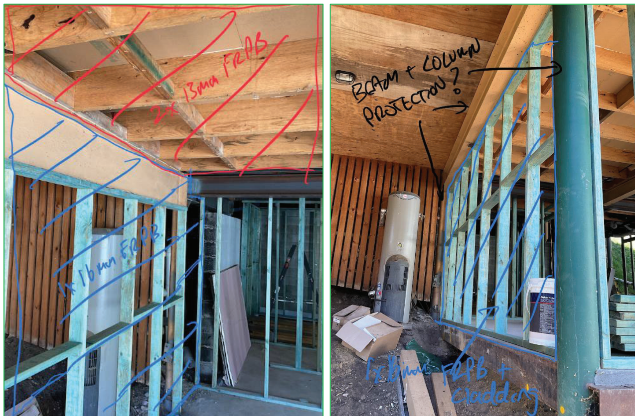
Figure 4-2 Undercroft separating wall non-continuous and exposed beams and columns over the allotment boundary.
