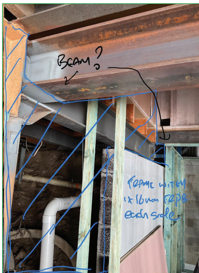
Figure 4-3 Beam penetrates through to adjacent dwelling's undercroft void.
